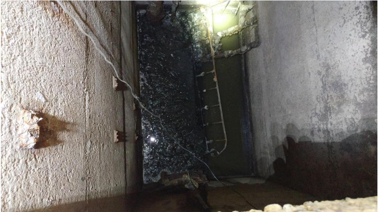
East Wet Well with Fallen Ladder Section
