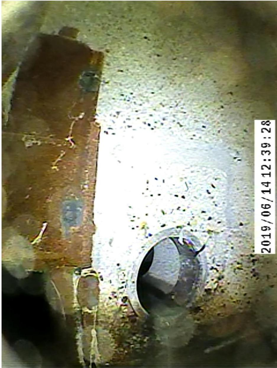
West Wet Well Looking at 600mm Diameter Inlet and 375mm Diameter Inlet Wastewater Pipes
